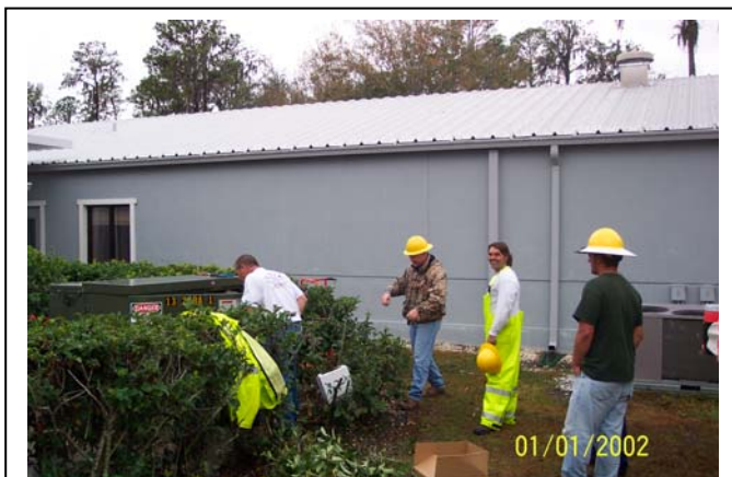
Peace River employees install new transformer.
